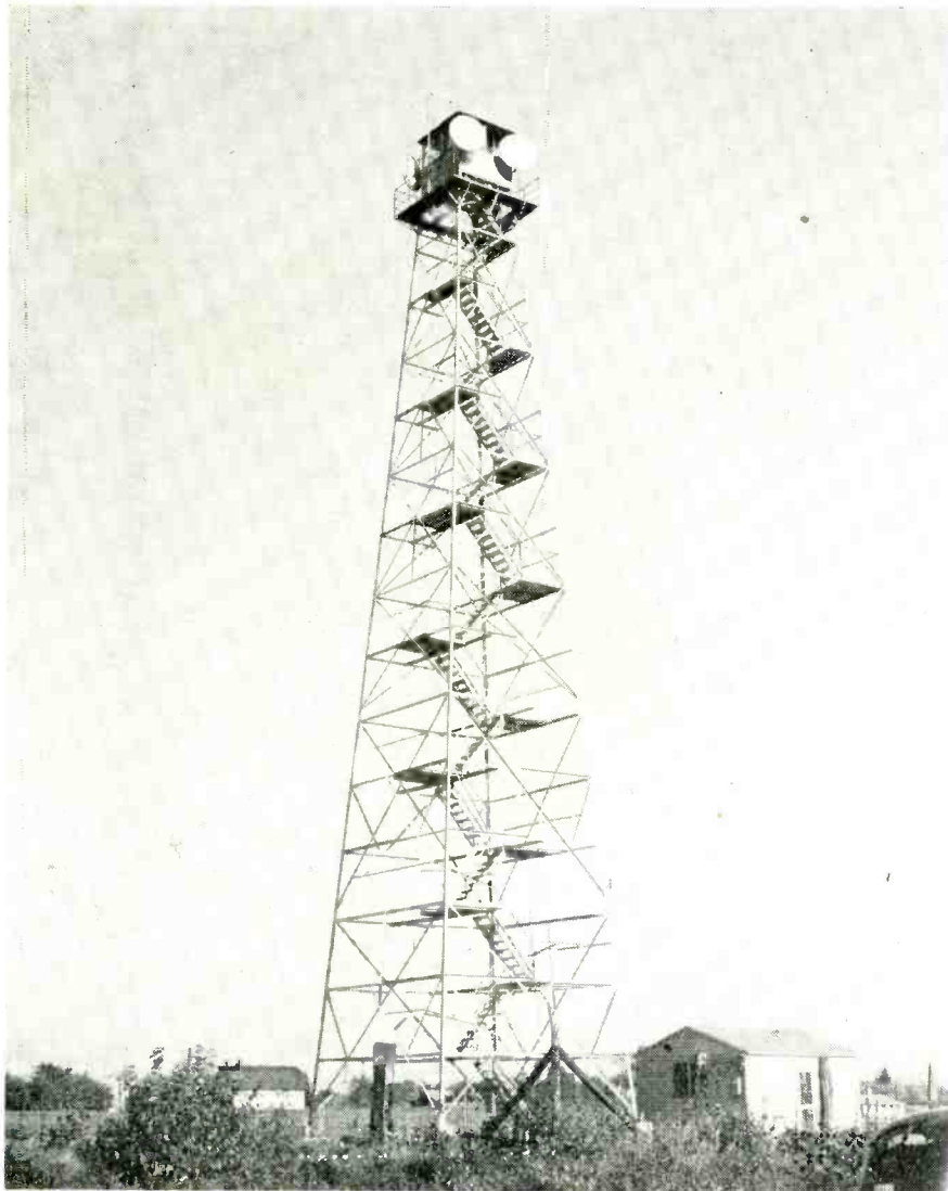
Relay Tower in RCA's New Microwave Communication System
